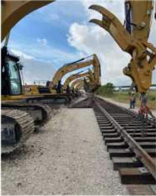
At the Rail Logistics project in Mont Belvieu, Texas existing track was demolished and a new #15 Turnout was installed.
